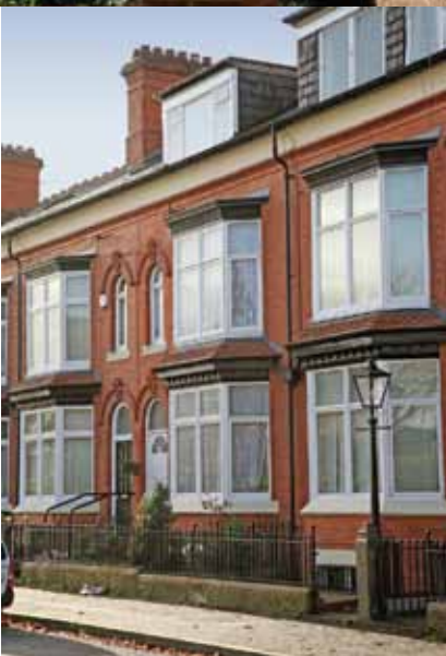
Social Housing refurbishment, Manchester
