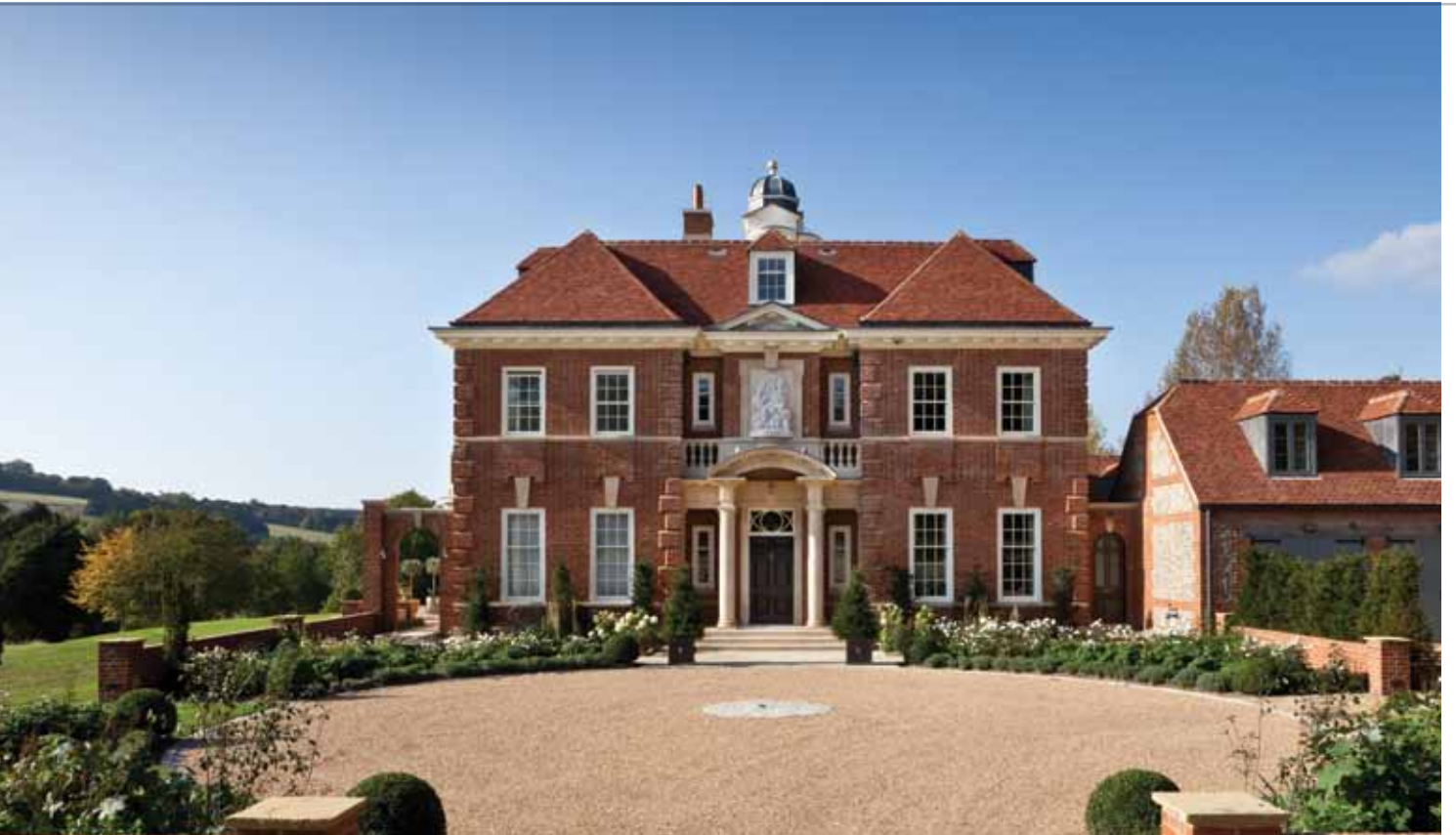
Prestige new build, Hampshire
