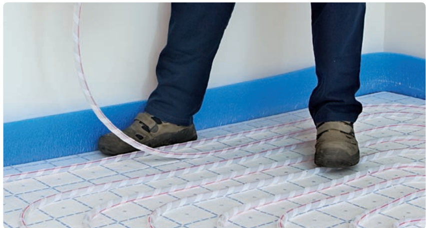
In case of misplacement, or if you want to straighten a line or tidy up just pull the pipe back up
