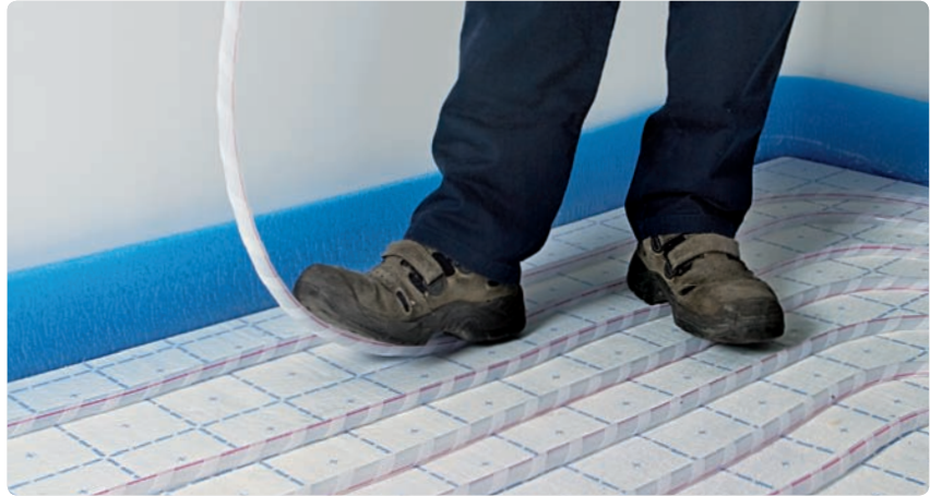
Simply tread on the pipe as you lay it in front of you. The pressure from your foot securely fixes the pipe in place
