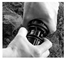
5. Nut Tightening The nut should be tightened by hand and then firmly with a wrench.
