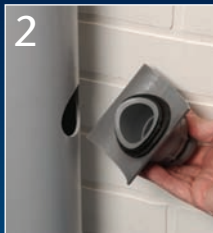
2 Ensure seal is in position
