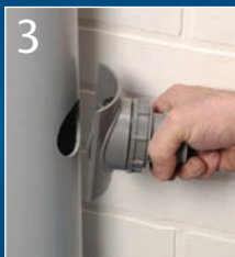
3 Insert Easy Boss into the hole
