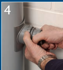
4 Twist in the Easy Boss connector
