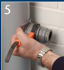
5 Use a strap wrench and hand tighten
