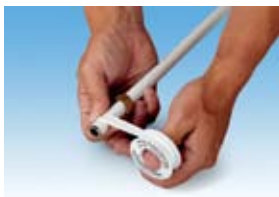
Apply PTFE tape if required
