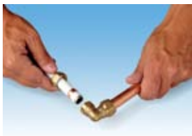
Ensure pipe is fully inserted
