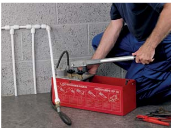
Fig. 57 Pressure testing
