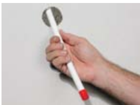
Fig. 22 Always protect pipe ends
