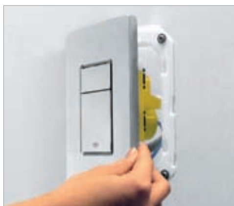
Open flush plate of the cistern with a fingertip.
