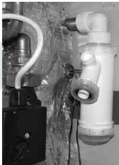
Figure 6-3: Condensate trap
