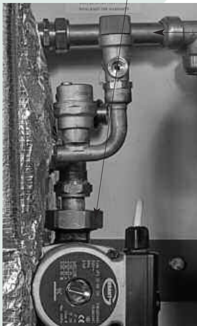
Figure 4-4: Removing flow & return pipe
