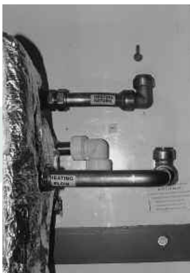
Figure 5-1: Non-system boiler flow and return connections
