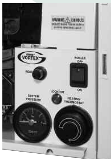
Figure 10-2: Boiler controls
