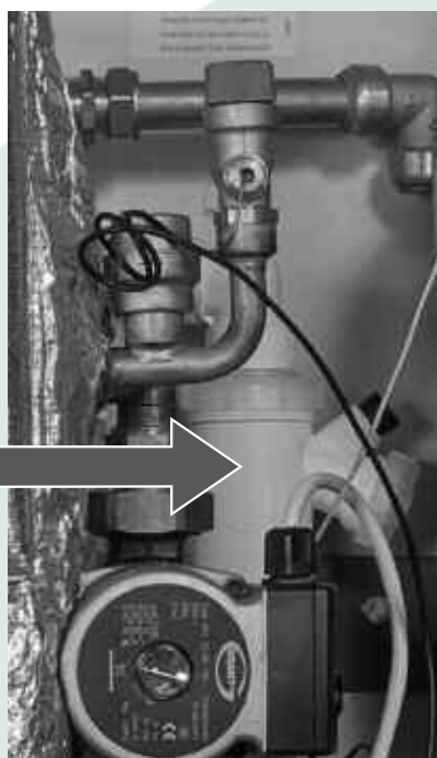
Figure 6-2: Condensate trap location in-situ
