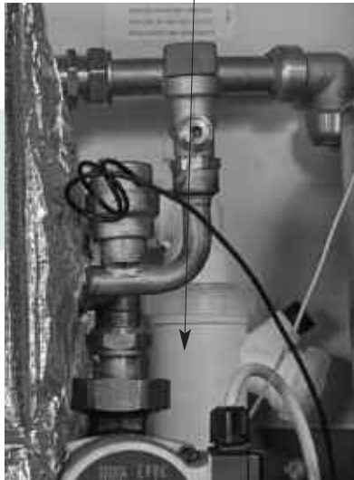
Figure 4-12: Re-fitting condensate trap
