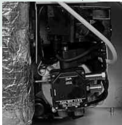
Figure 4-5: Removing burner
