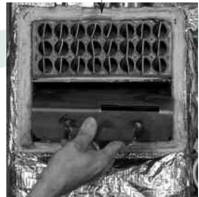
Figure 4-7: Removing baffles from boiler shell
