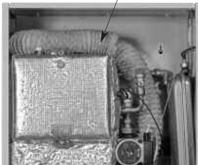
Figure 4-13: Re-fitting snorkel tube
