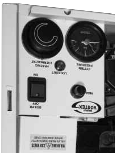
Figure 2: Boiler controls
