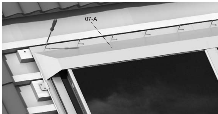
Figure 73: Fixing left hand Top Cover Flashing (07-A)
