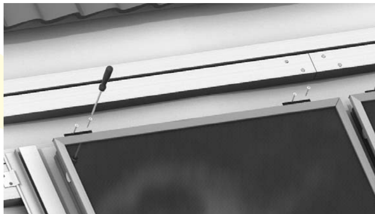
Figure 71: Fixing of the Top Brackets
