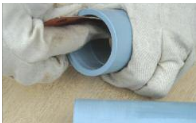
4. Abrade pipe and fitting.
