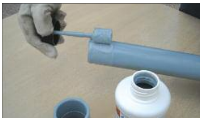
9. Apply cement to pipe and fitting.
