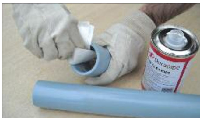
7. Clean pipe and fitting with eco cleaner.
