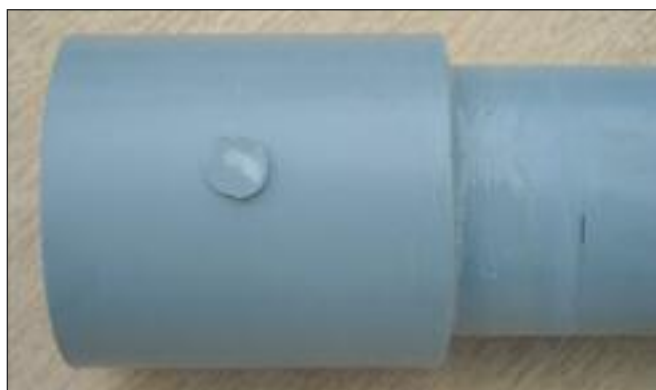
12. Using the previously marked guide, check the pipe is fully inserted into the fitting.
