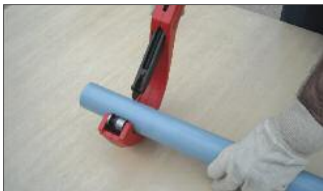
2. Cut pipe to required length.
