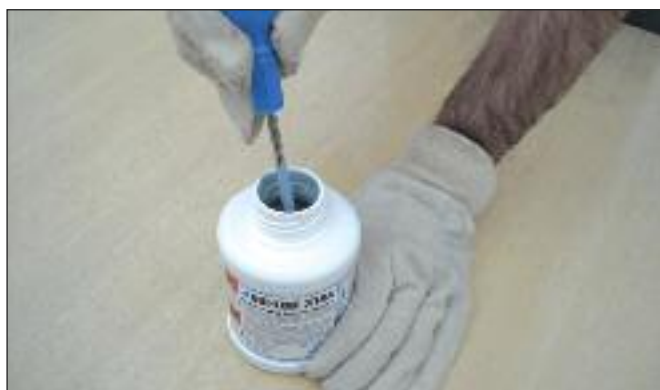
8. Stir solvent cement.
